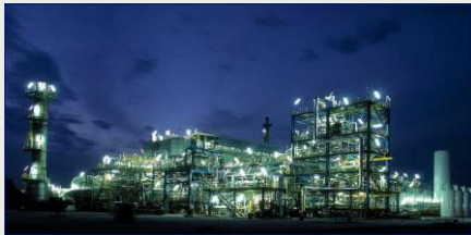
Air Liquide, Port Jerome (SMR +CCS)
