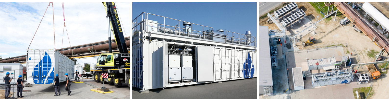
Left: Electrolyser installation at the Salzgitter Flachstahl steel plant (© Salzgitter AG); Middle: Sunfire-HyLink SOEC electrolyser (© Sunfire GmbH); Right: Drone shot of the GrInHy2.0 installation at the Salzgitter Flachstahl steel plant (© Salzgitter AG)
